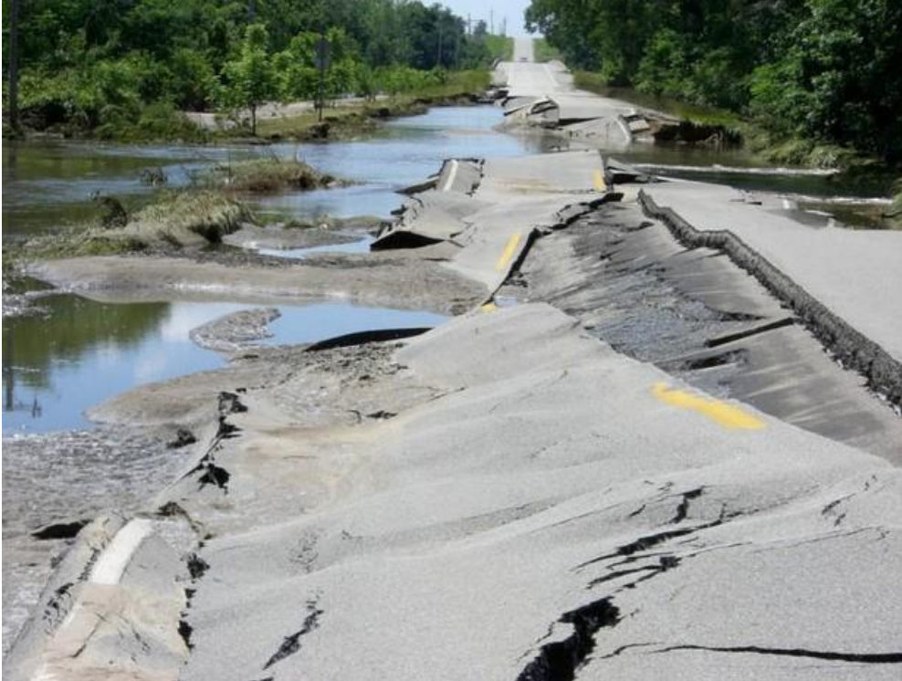
Figure 8. Significant damage to U.S. Highway 6 becomes apparent after the Cedar River subsides east of Atalissa, Iowa in June 2008. Photo by the Iowa Department of Transportation.
